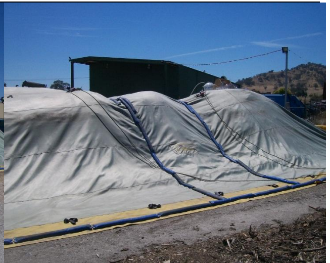
First and second heap separated with inert buffer material
